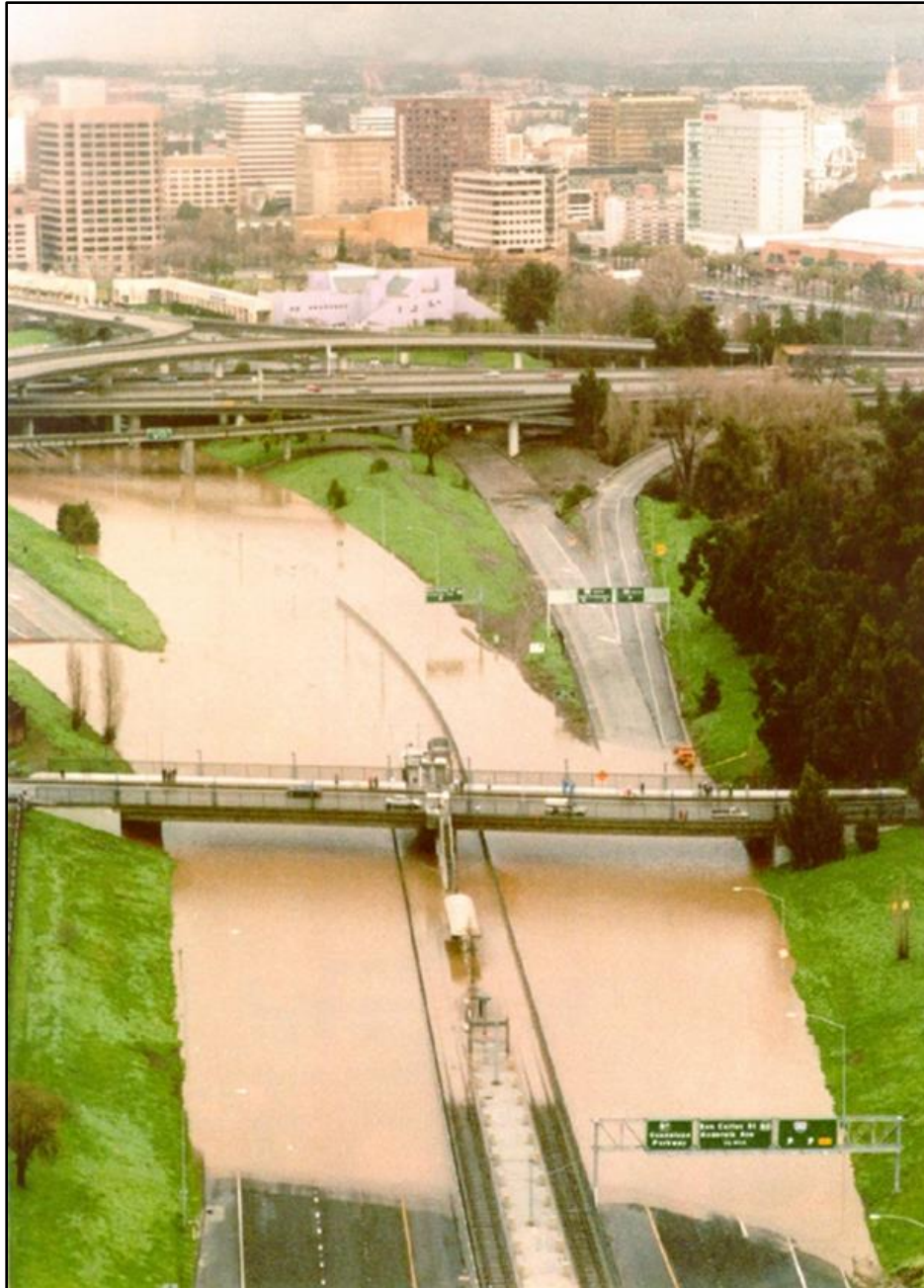
Figure 5. Photograph of flooding in the Flood of January 9, 1995. Downtown San José is seen in background. (Source: Valley Water)
